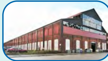
1310 East Ave_Erie City Iron Works
