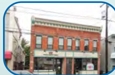
1310 East Ave_Erie City Iron Works
